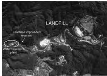
Photo 4.3 Aerial view of garbage dumped landfill and facilities.
